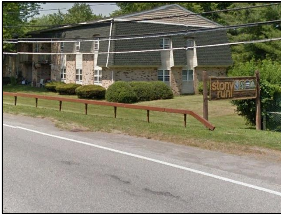
Existing box beam guide rail
