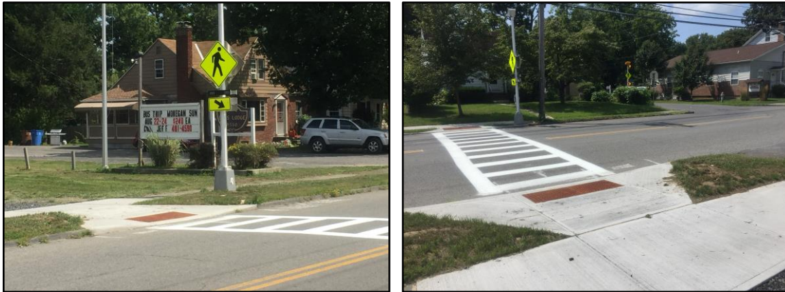
Mid-block crossing east of Quarry Street with LED pedestrian crossing equipment
