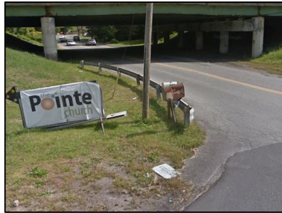
Existing W-beam guide rail
