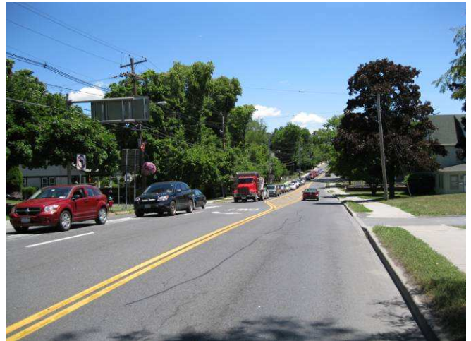
Main Street, New Paltz, Looking East at Westbound
