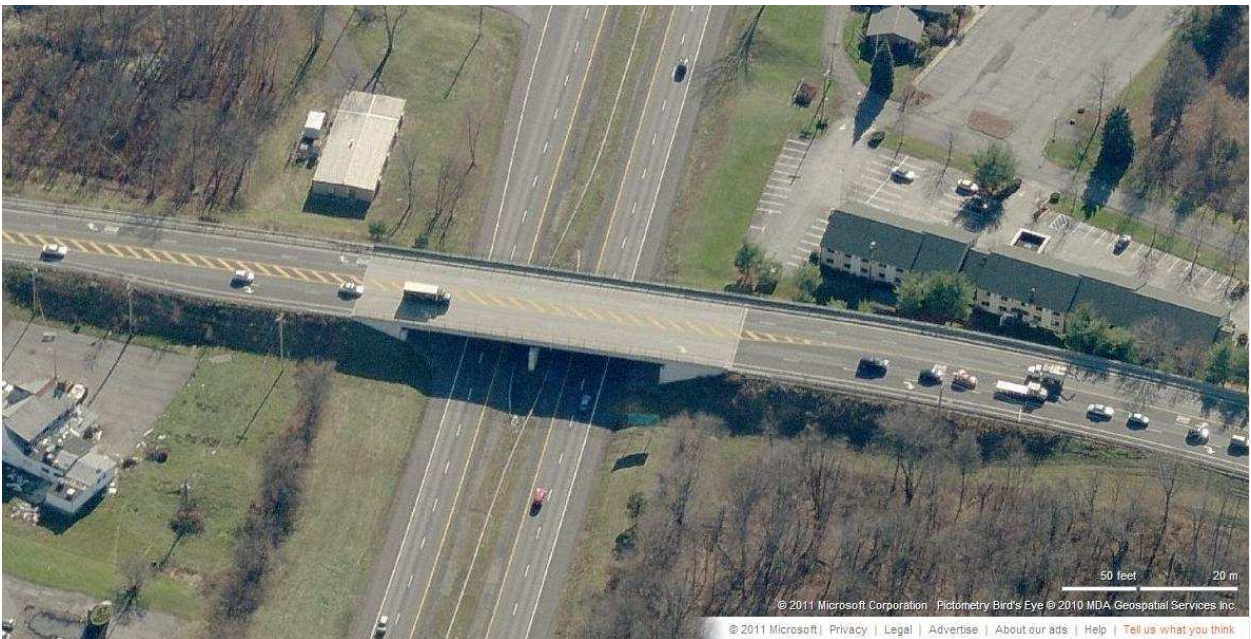
Aerial Perspective of the NYS Route 299 Thruway Bridge. The north façade is visible.
