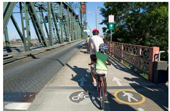
Bridge Shared Path and Markings
