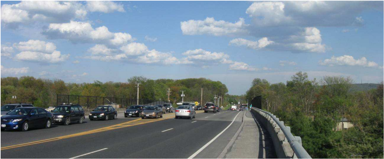
Route 299 - NYS Thruway Bridge looking east
