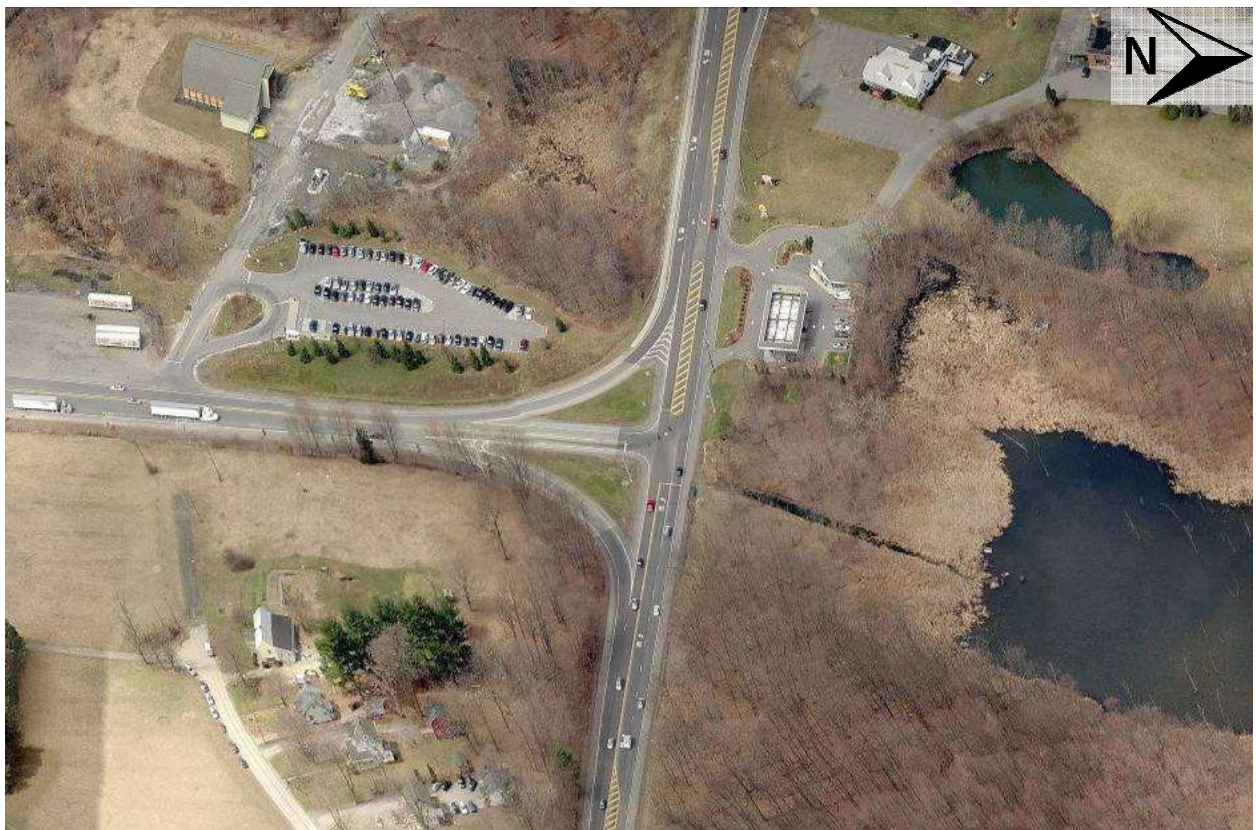
Intersection of NY 299 with Thruway (I-87) Interchange
