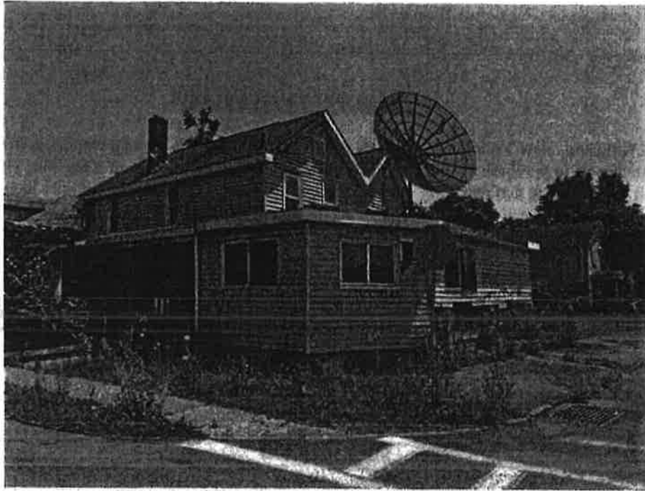
Figure 2 - 46 Grand Corner Grand St/Hasbrouck Avenue
