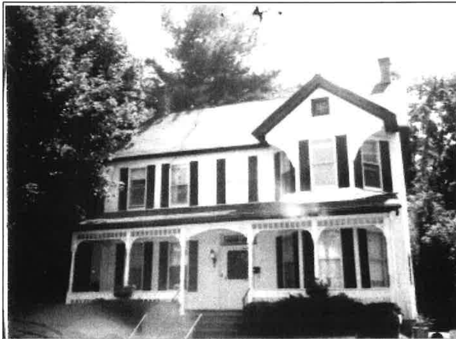
Figure 6: Circa 1960s photograph of 54 W. Chester Street. Courtesy of the City of Kingston's Assessor Office, 2024.
