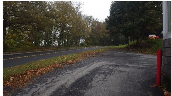
Photograph #2 – Sight Distance Looking Right
