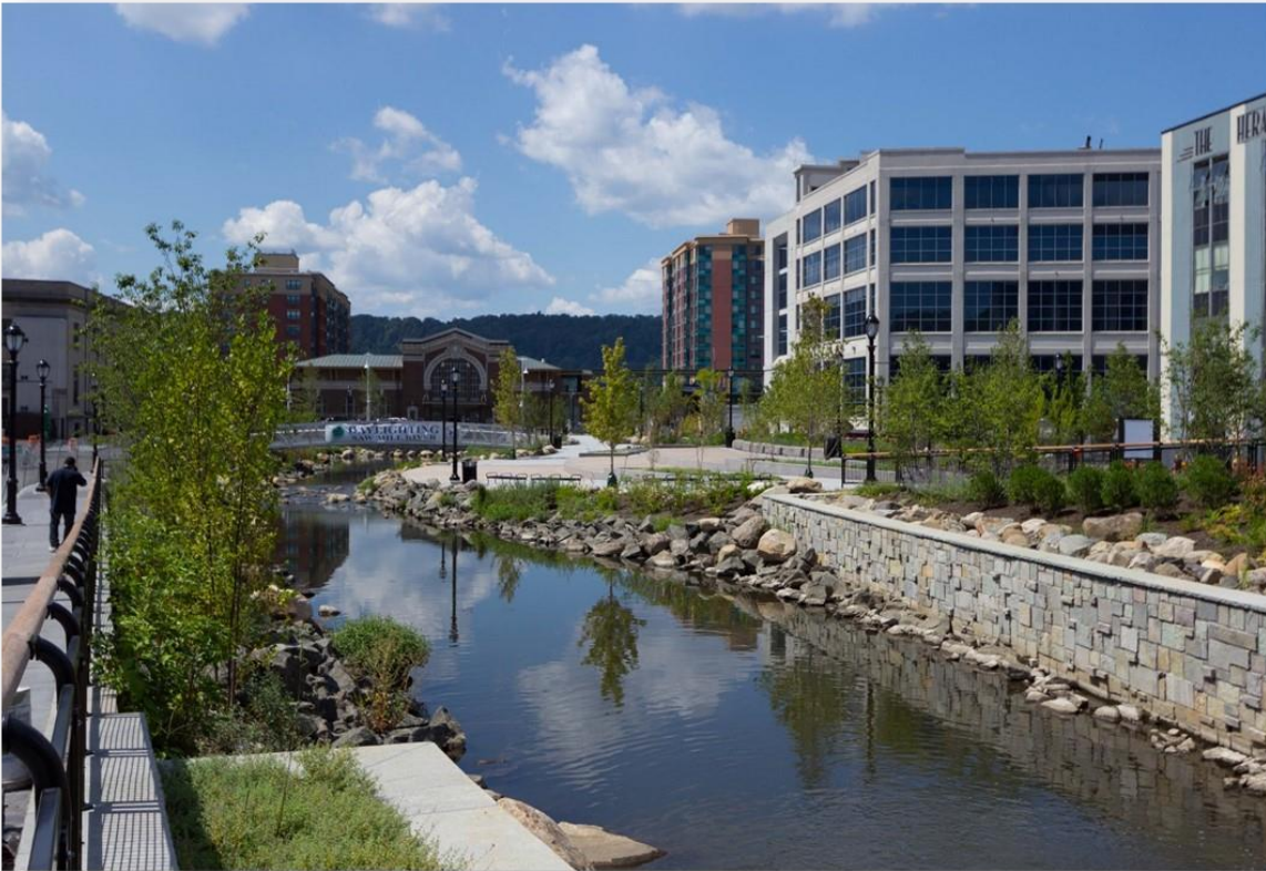
Figure 3. Daylighting of the Saw Mill River in Yonkers, NY. Credit: NYS Environmental Facilities Corporation
