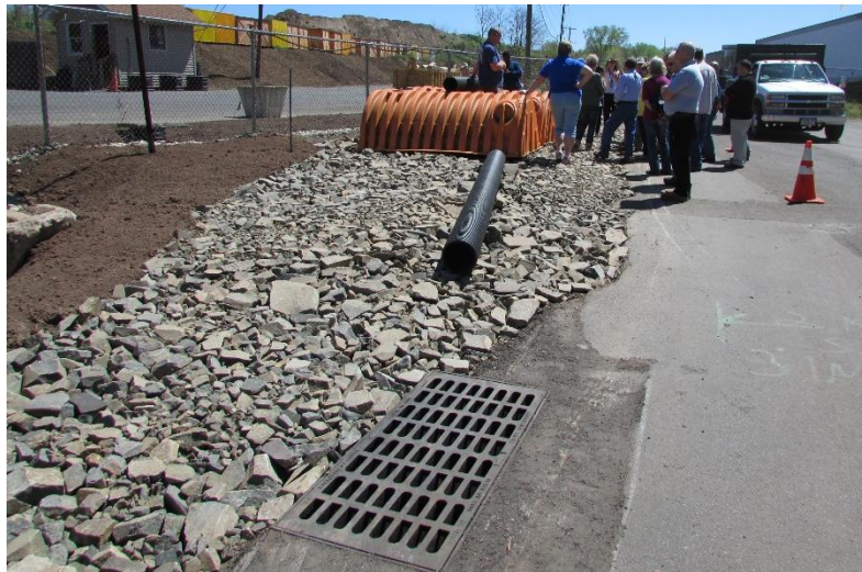
StormChamber, Orangetown Highway Department
