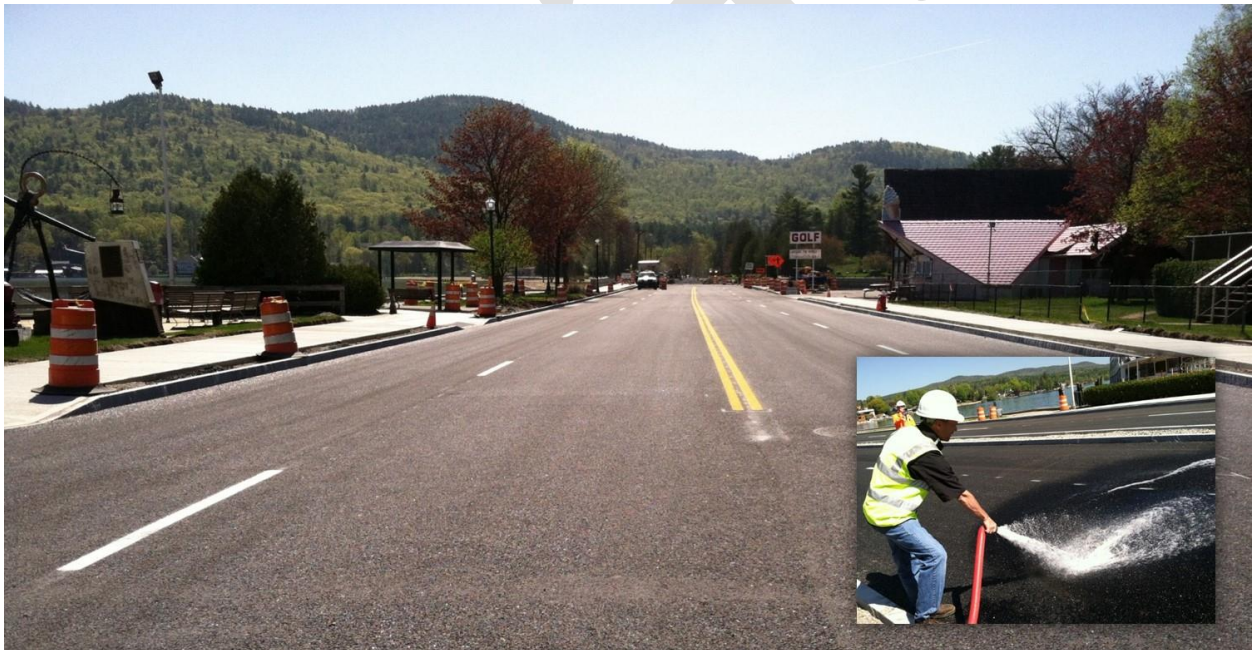
Figure 6. Porous pavement and a demonstration of infiltration in Lake George, NY Credit: NYS Environmental Facilities Corporation
