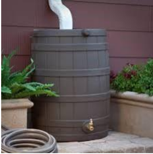
Figure 5. Rain barrel capturing rooftop runoff. Credit: NYS Environmental Facilities Corporation
