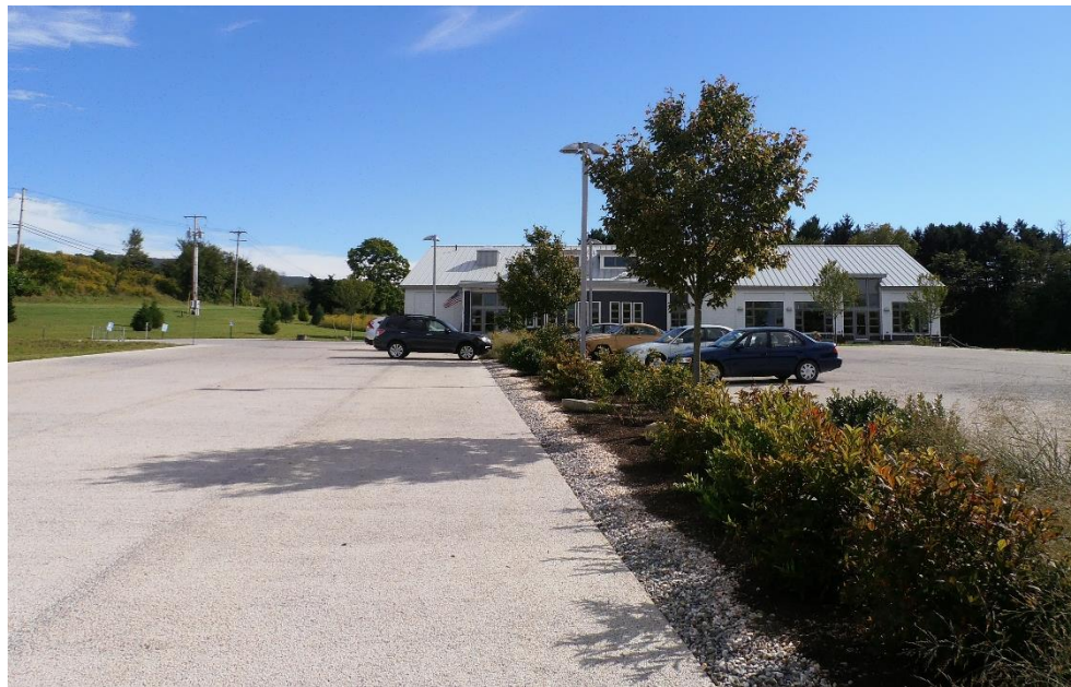
Pervious Pavement and Vegetated Swale, Roeliff Jansen Community Library
