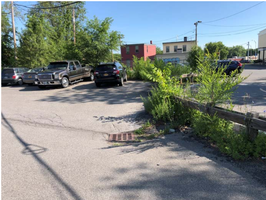
Drainage structure located along edge of parking lot
