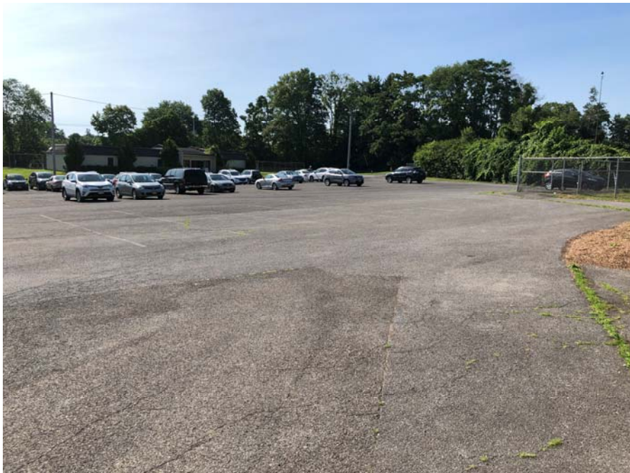
Overall picture of parking area
