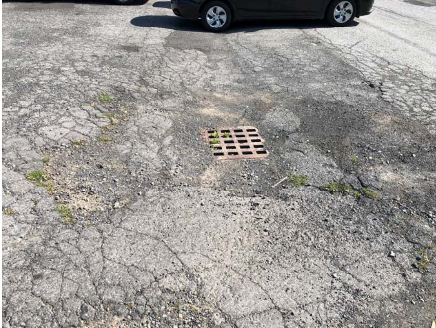
Picture of drainage structure in parking lot along Severyn Street
