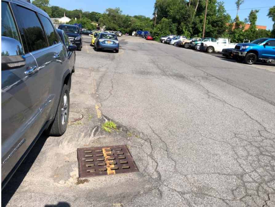
Drainage structure located adjacent to drive isle
