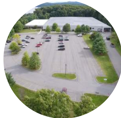
Live next to industrial units. Do all necessary interventions that can allow the development of quality housing next to industrial units.
