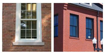
Figure 405.14.E.2.b: Sills. Cast Concrete (left) and Brick (right)
