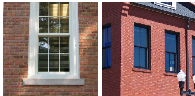
Figure 405.14.E.2.b: Sills. Cast Concrete (left) and Brick (right)
