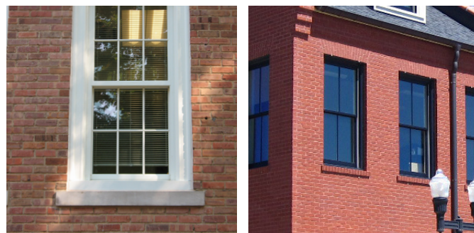
Figure 405.14.E.2.b: Sills. Cast Concrete (left) and Brick (right)
