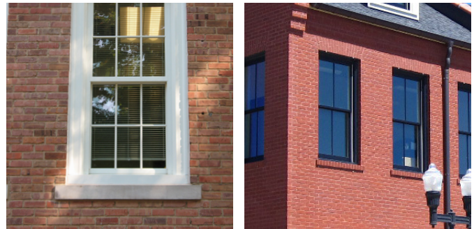
Figure 405.14.E.2.b: Sills. Cast Concrete (left) and Brick (right)
