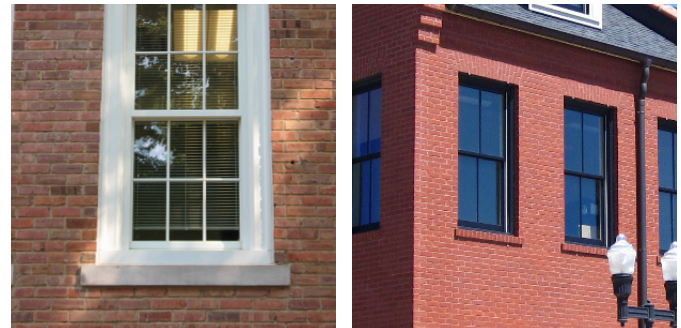
Figure 405.14.E.2.b: Sills. Cast Concrete (left) and Brick (right)
