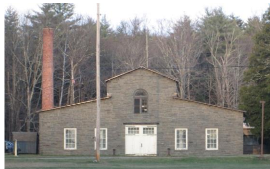
Edmund T. Cloonan Water Treatment Plant
