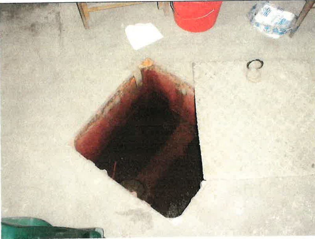
Existing access door in basement floor – original sanitary piping passes through
