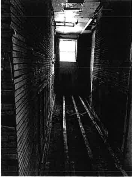
2 nd floor Work Area (Post-Abatement)
