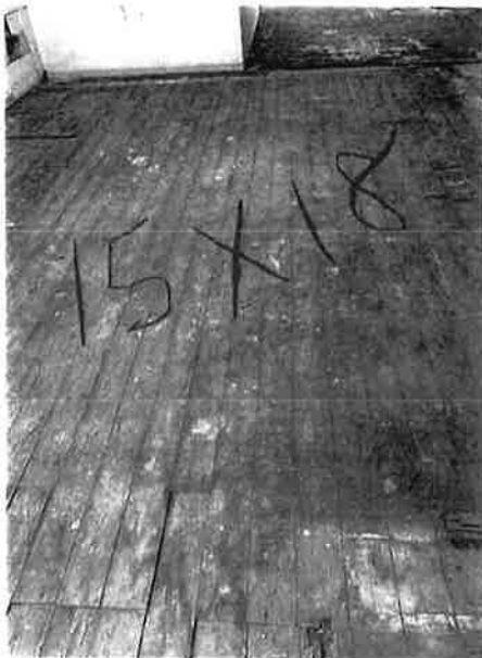
(Left) 15x18 Mastic on top of nailed plywood
