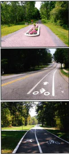
**Above** (top to bottom): Gateway to dedicated rail trail, which is a multi-purpose trail; example of an on-street painted bike path and an off-Street combination sidewalk/bike path.
