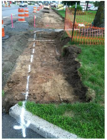
**Figure 36.** Protecting existing trees appropriately when doing needed construction. Utilization of structural soil for street tree plantings along sidewalks and other paved areas allows installation of hardscape features such as concrete or bluestone walks and granite curbs without damage from healthy tree root growth. Underneath the tree in the image below is a large bed of CU ™Structural Soil extending several feet in either direction around and below the root ball.
