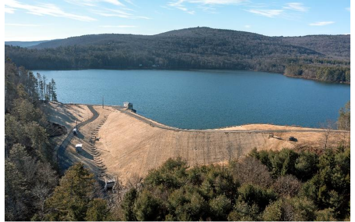
Dam at Cooper Lake Reservoir
