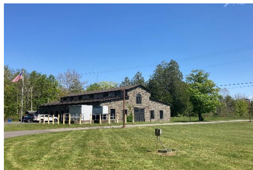
Edmund T. Cloonan Water Treatment Plant
