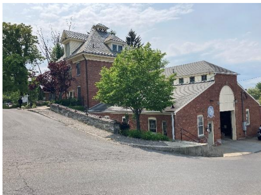
111 Jansen Ave Building
