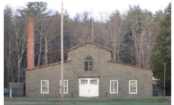
Edmund T. Cloonan Water Treatment Plant
