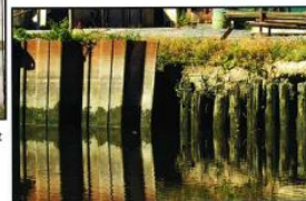
Photo 44 - Steel Sheet Piling and Vertical Timber Piles
