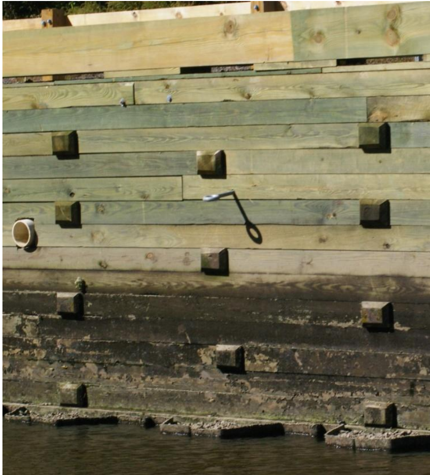
Figure 17 - Timber Bulkhead
