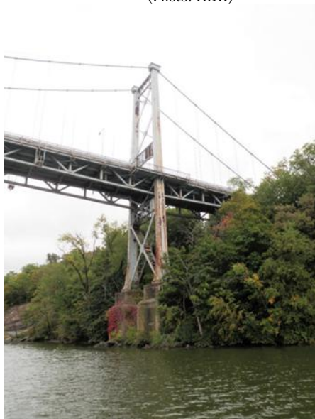
Photo 5 – Port Ewen Suspension Bridge (Photo HDR)
