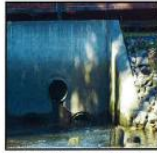
Photo 13 - Concrete Culvert and Small Rip Rap, Timber Cribbing, Concrete wall with Concrete Slabs
