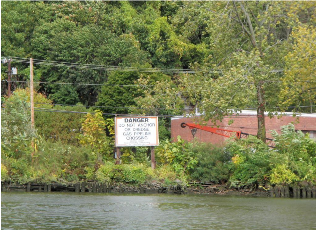
Photo 50 - Pipeline Crossing (Photo: HDR)
