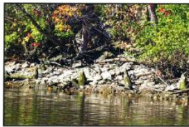
Photo 41 - Unprotected Shoreline with Abandoned Commercial Piers
