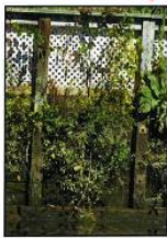
Photo 29 - Horizontal Timber Cribbing with Timber Fenders
