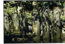
Photo 34 - Timber Cribbing with Timber Piles and Rope
