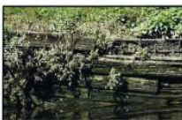
Photo 26 - Timber Cribbing in Fair to Poor Condition
