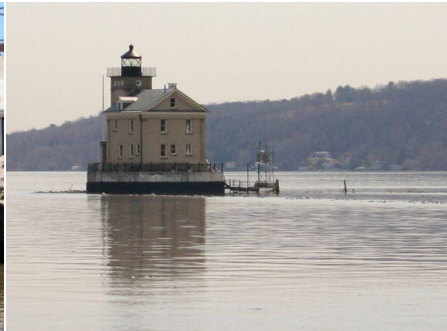
Photo 47 – Submerged Jetty (Photo: www.kingstonlighthouse.com)
