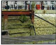
Photo 9 - Steel Frame with Timber Cribbing and Precast Concrete Blocks
