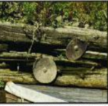
Photo 17 - Timber Cribbing and Piles with Timber Fenders
