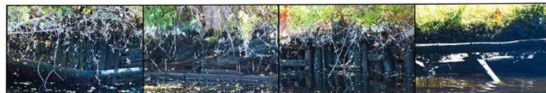
Photo 27 - Various Forms of Timber Cribbing and Piles in Disrepair with Loose Connecting Rods and Erosion
