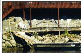
Photo 42 - Large Stone with Dock Supports and Building Foundations
