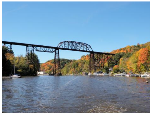
Photo 6 – West Shore Railroad Trestle (Photo: HDR)
