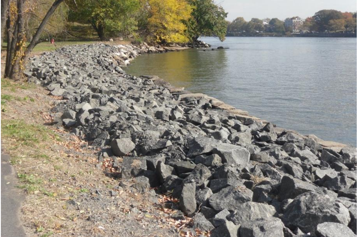
Figure 14 - Rip rap (Photo: Randall's Island Seawall Stabilization – HDR)
