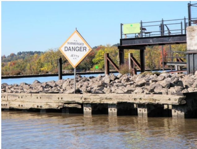
Photo 46 – Submerged Jetty Sign (Photo: HDR)
