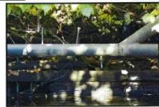
Photo 33 - PVC Pipe atop Horizontal Timber Cribbing with Exposed Connecting Rods
