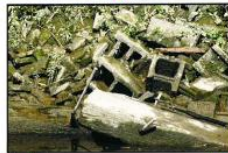
Photo 32 - Masonry Blocks and Rip Rap
