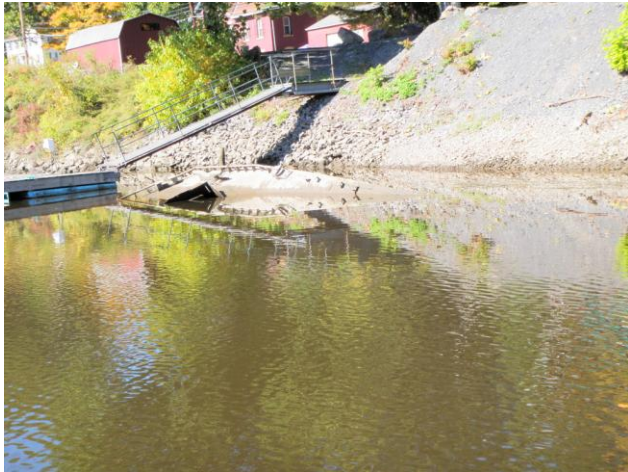
Photo 48 – Submerged Steel Deck Barge (Photo: HDR)
