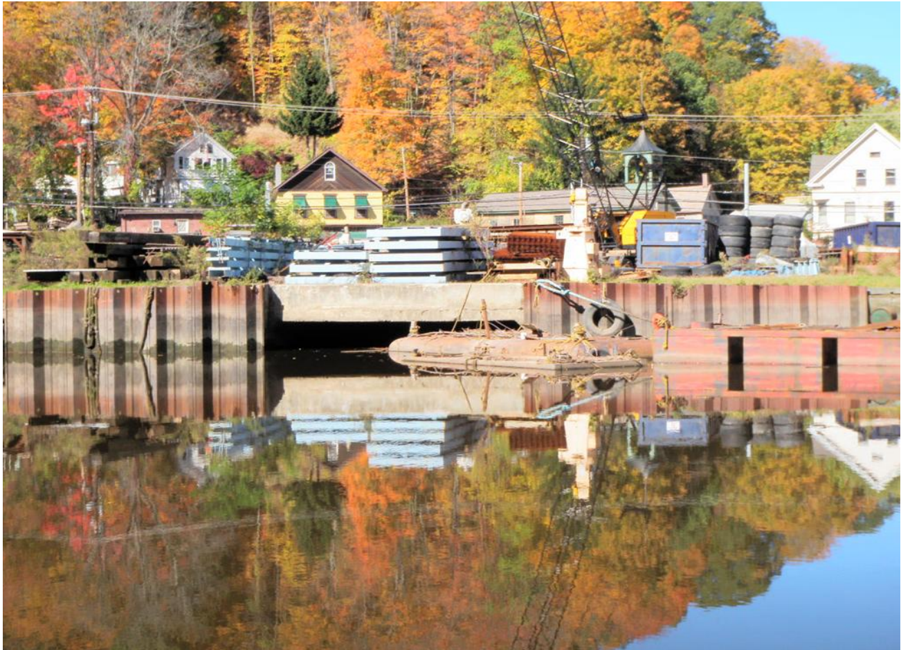
Photo 51 – Twaalfskill Brook Outfall (Photo: HDR)
