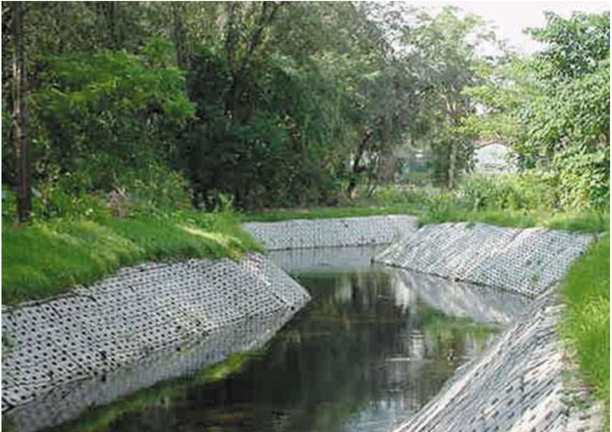
Figure 15 - Articulated Concrete Block (Photo: landandwater.com)
