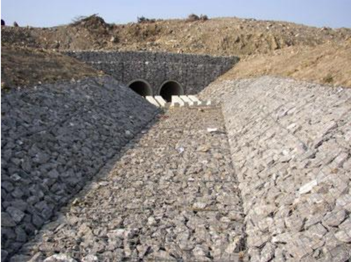
Figure 16 - Gabion Baskets (Photo: ridgeway-online.com)
