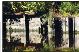
Photo 43 - Sheet Metal with Soldier Piles and Steel Sheet Piling
