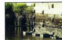
Photo 28 - New Timber Bulkhead (2010)
