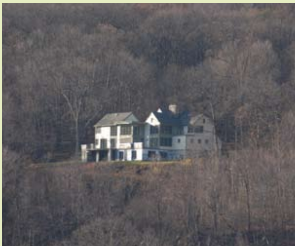
Even with provisions of Waterfront Bluffs Overlay District, this home still lies unshielded from river.
