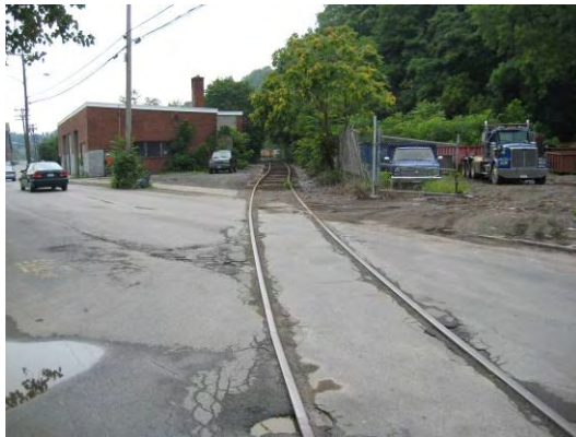
Figure 13 – track alignment east of car yard
