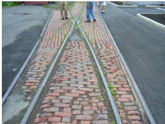
Figure 25 – Brick pavers broken in various configurations
