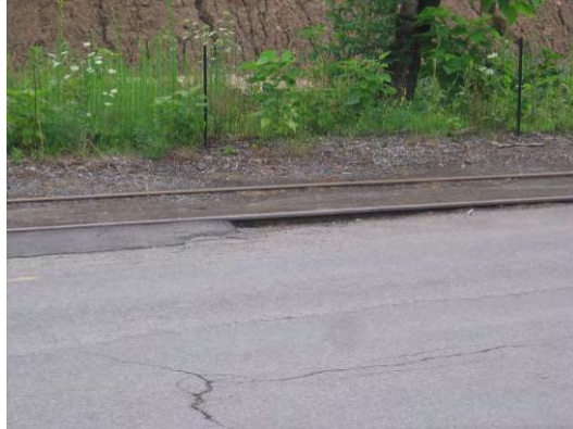
Figure 27 – East Strand roadway track interface
