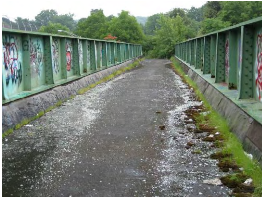
Figure 326 – on bridge over Route 9W looking east
