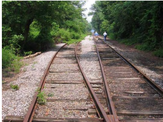
Figure 6 – at west end of siding track looking east
