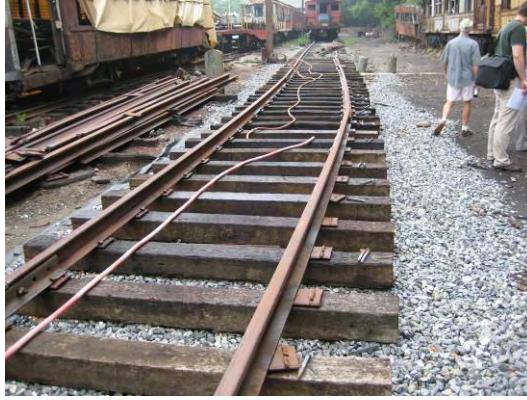
Figure 9 – Car yard skeleton track
