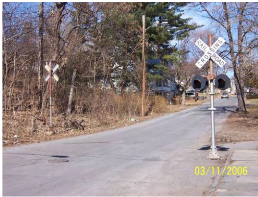
Figure 61 – Removed Crossing Flashers at 1 st Avenue
