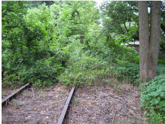
Figure 38 – Overgrown ballast between Delaware Ave and Elm St.
