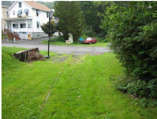
Figure 51 – Rails paved over and grown over at 2 nd Ave Grade Crossing
