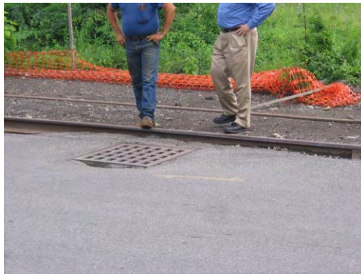
Figure 28 - Drainage Manhole adjacent to track on East Strand
