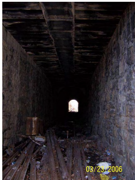
Figure 45 – Stockpiled rail inside rail tunnel
