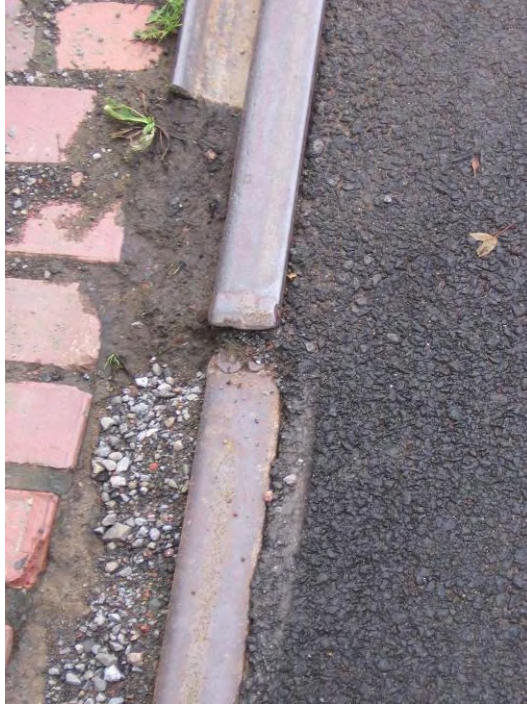
Figure 24 – Rail end mismatch and broken flangeway of girder rail in embedded track
