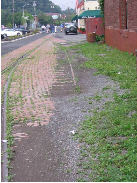
Figure 18 – Two embedded turnouts east of museum looking west along E. Strand
