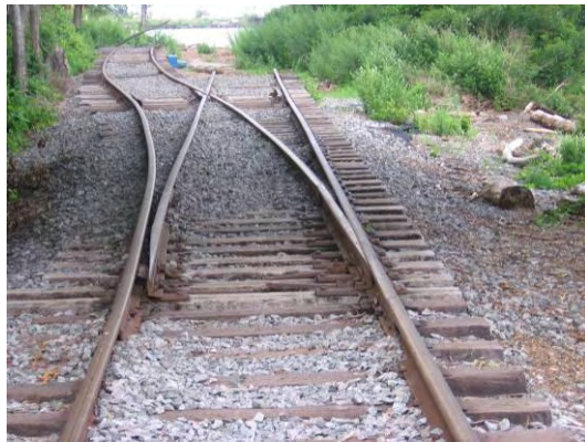
Figure 23 – Turnout at Kingston Point
