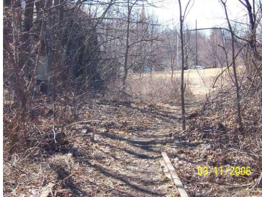
Figure 53 – Rails removed at second Delaware Ave grade crossing
