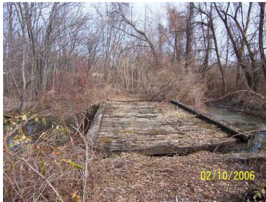
Figure 57 – Northernmost open deck bridge along west side of lagoon
