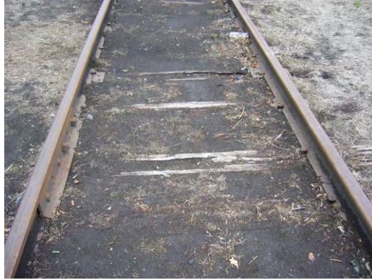
Figure 15 – Fouled ballast near Kosco
