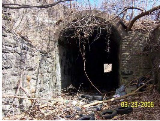
Figure 44 – Approach to north side of rail tunnel
