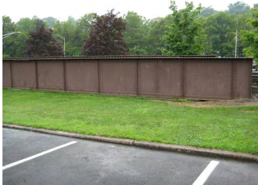
Figure 60 – Retaining wall adjacent to single span open deck bridge along Rondout Drive
