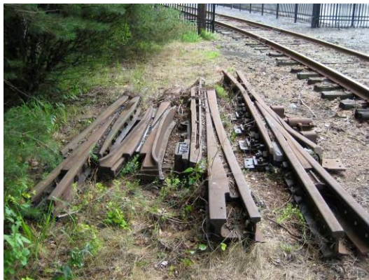
Figure 17 – Stockpiled turnout parts at car yard
