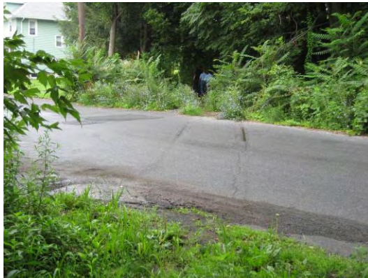
Figure 52 - Rails partially paved over at 1 st Ave Grade Crossing
