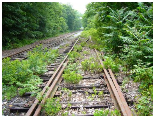
Figure 34 – Kingston Point Line siding track looking west at turnout to Brickyard spur track
