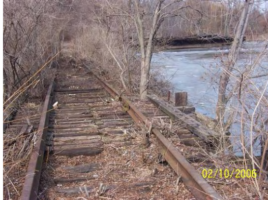
Figure 56 – Middle open deck bridge along west side of lagoon
