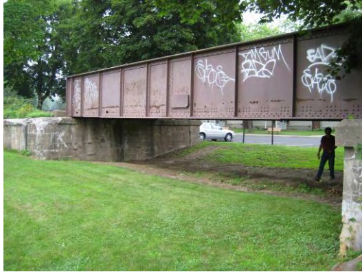
Figure 59 – Clearance under southernmost railroad bridge along Rondout Drive
