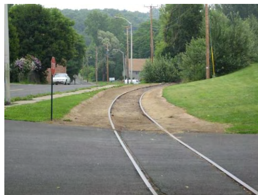
Figure 46 – Grade Crossing at Maple Street
