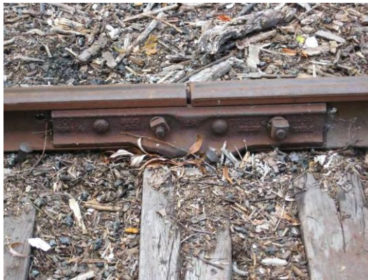
Figure 10 – Compromise Joint Bars connecting 80# and 105# Dudley rail
