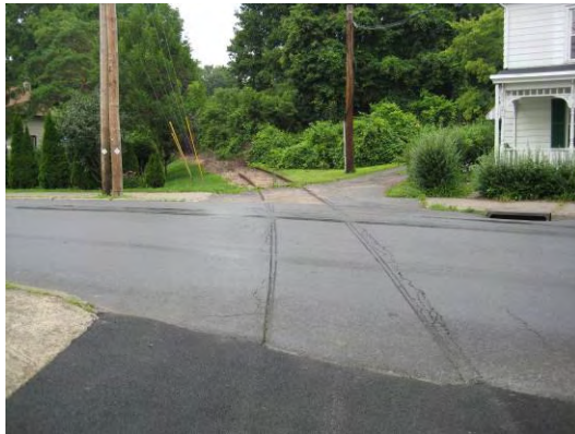
Figure 48 – Rails paved over at Delaware Avenue Grade Crossing
