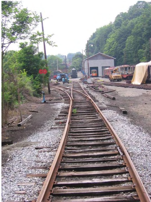
Figure 21 – No. 8 Turnout to West Strand Crossing (left)
