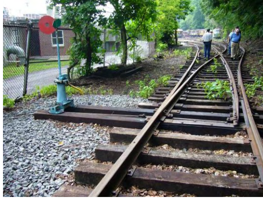
Figure 20 –No. 8 Turnout from Mainline to Yard / Shop Lead
