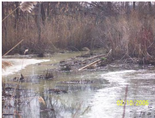
Figure 58 – washed away track roadbed south of Delaware Ave west side of lagoon
