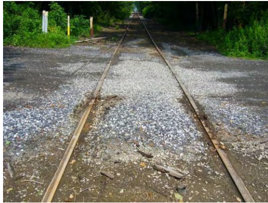
Figure 5 – at North St. extension looking east toward causeway with gas line marker on far side of crossing
