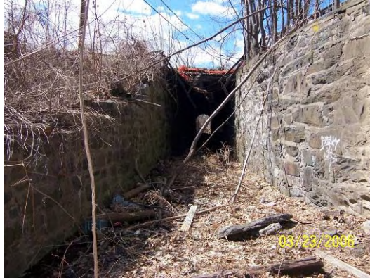
Figure 33 – looking west toward tunnel beneath Livingston St., Hasbrouck Ave., and Delaware Ave.
