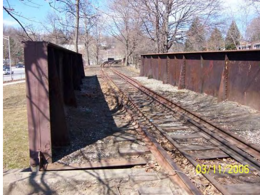
Figure 41 – Ballasted deck bridge along Rondout Ave closest to museum
