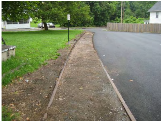
Figure 49 – pavement to field side of one rail on section of track between Murray St. and Delaware Ave
