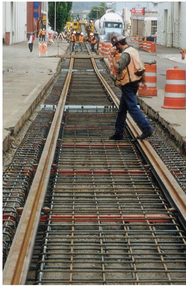
Figure 67 - Girder Rail Track Construction
