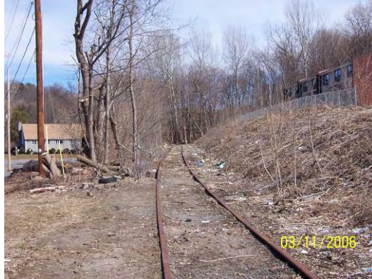
Figure 37 – fouled ballast north of Maple Street
