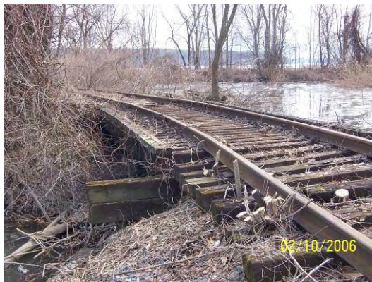
Figure 55 – Southernmost open deck bridge along west side of lagoon
