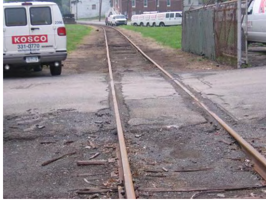
Figure 4 – near Kosco looking west toward E. Strand
