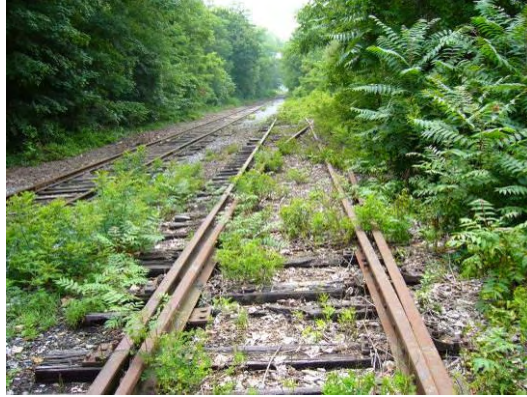
Figure 7 – on siding track looking west at turnout to Brickyard spur track
