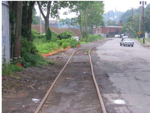
Figure 14 – Variable Gauge along E. Strand east of museum
