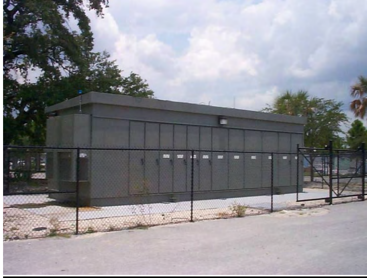
Figure 68 – Typical Streetcar Substation
