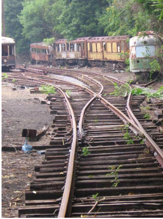
Figure 22 – Yard Lead Track Turnouts
