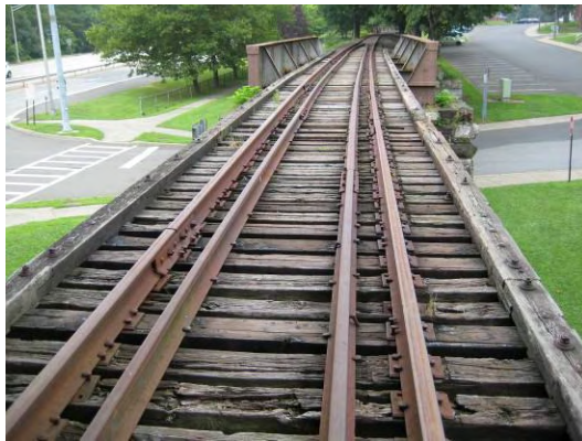
Figure 42 – Three span open deck bridge over Garraghan Drive
