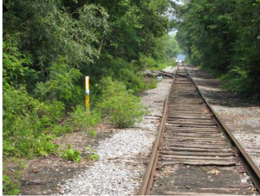
Figure 30 – Gas line marker at east end of siding looking east toward causeway
