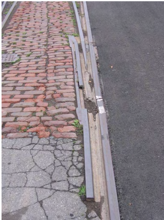
Figure 19 – Embedded Turnout on E. Strand
