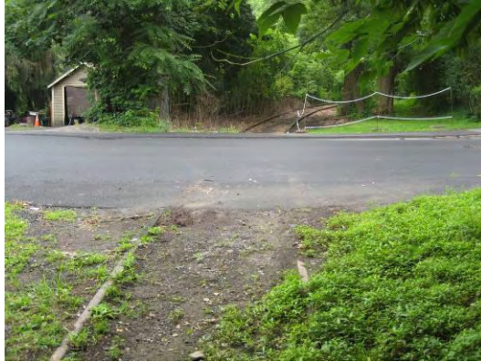
Figure 50 – Rails paved over at Elm Street Grade Crossing
