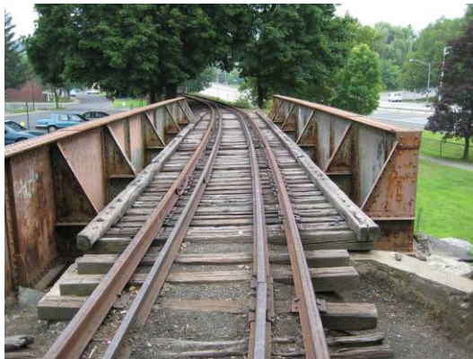
Figure 43 – Single Span open deck bridge north of Garraghan Drive
