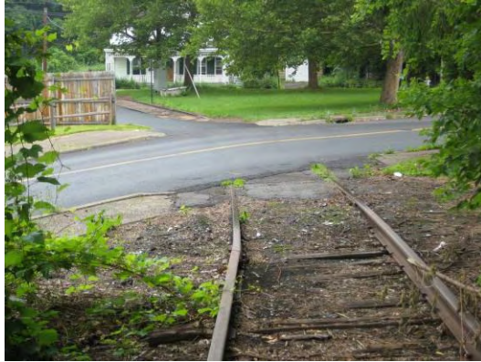
Figure 47 – Rails paved over at Murray Street Grade Crossing
